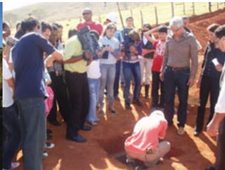
Placing the time capsule and cornerstone at the school groundbreaking ceremony
